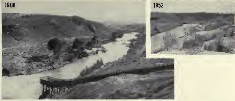
CONCRETE REPLACED WOODEN STRUCTURES. The number of irrigated acres increased from 20,784 in 1906, to 46,085 in 1928 and 58,893 in 1950. At left the old wooden chute from Truckee Canal (photo by S. R. Moreon). Inset, Lohontan Dam and Power Plant. Photo by H. Smith Richards, Region 4 engineer.
